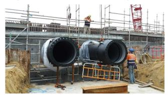
Ductile cast iron ball type flexible expansion joint called TAI-FLEX (size DN 1000mm) were installed at passenger clearance terminal located at Hong Kong-Zhuhai-Macau Bridge. Building constructed on an artificial island experience land subsidence, and Tai-Flex was chosen to protect the water pipeline.
